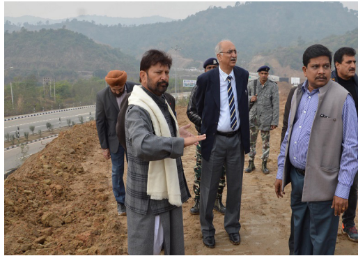
Development works being executed by the
